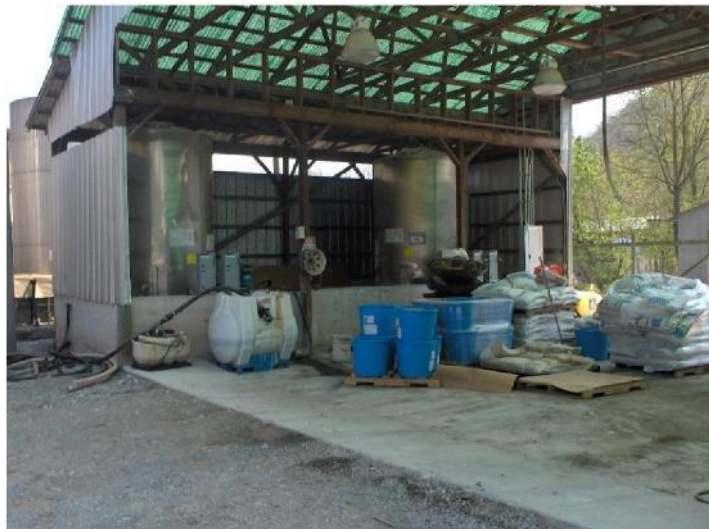
Secondary containment at a bulk pesticide facility
