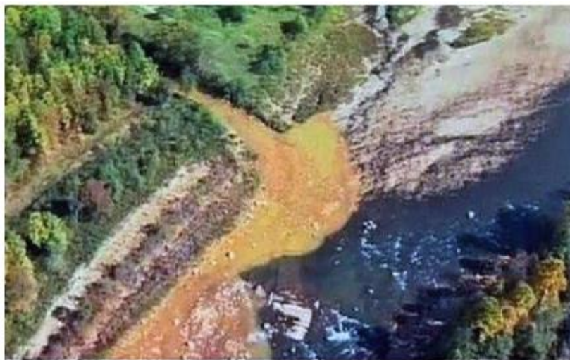
Aerial photo 1994 Mine Blowout - Photo Credit Randy Robinson
