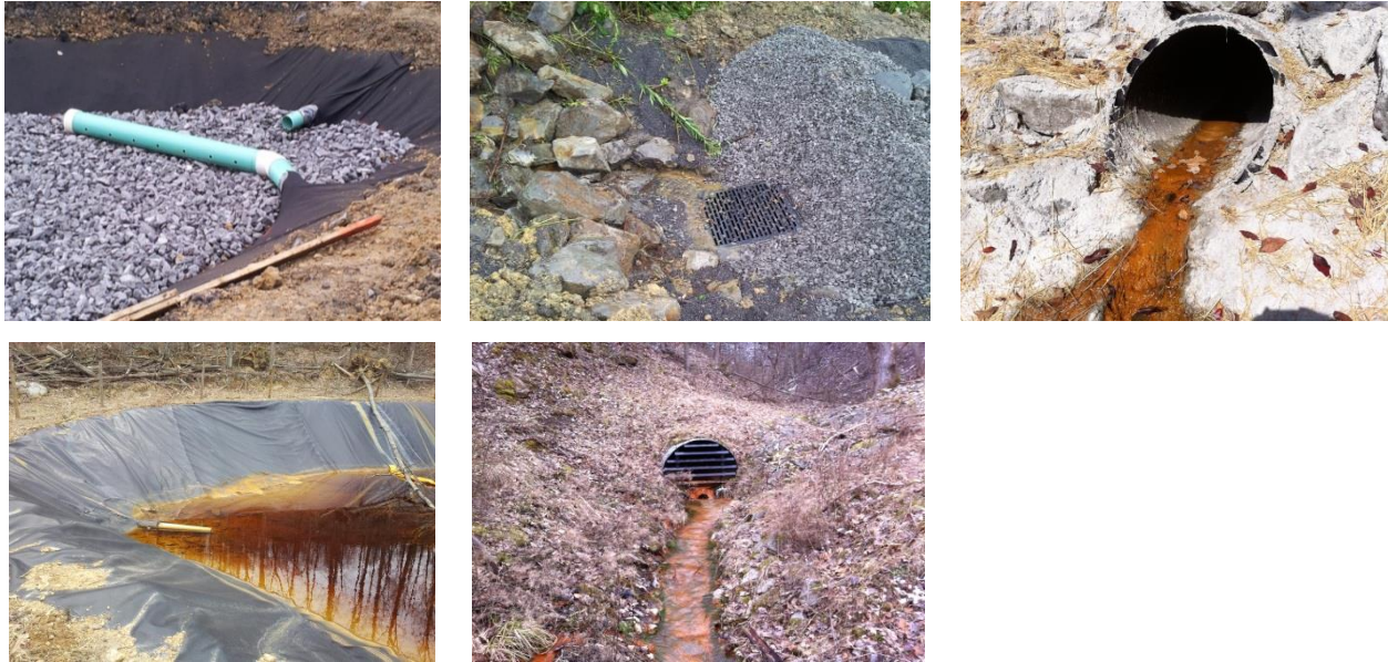
Figure 5: BMPs where flow is difficult to measure, including pipes discharging water through multiple perforations; a drop inlet from a channel, a pipe into a grouted channel with no lip beneath the pipe, an inlet pipe submerged beneath the surface of a pond, a transition from a bat gate to an open limestone channel.
