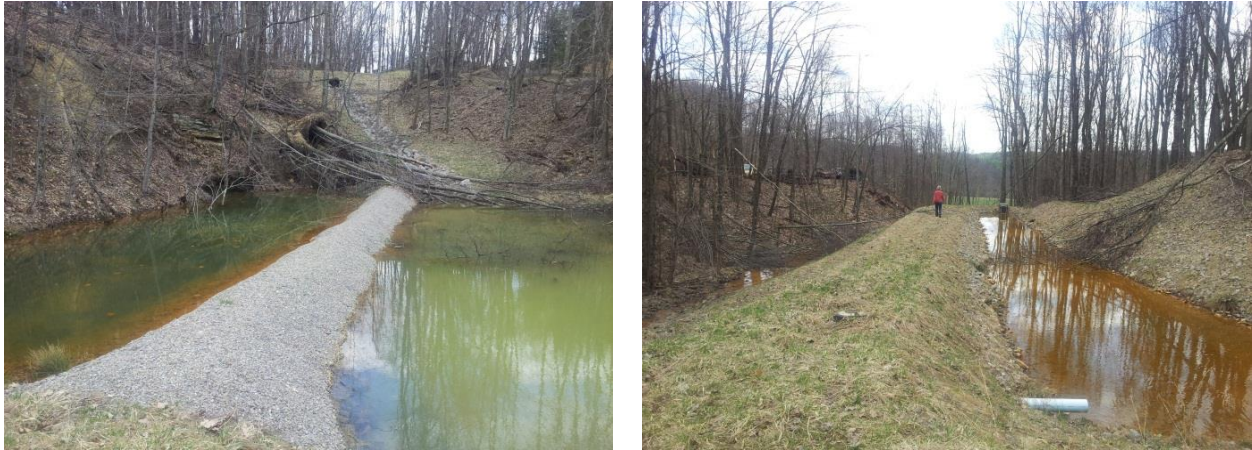
Figure 13: Operation: Adjust the mixture of water from an AMD source with water from a steel slag leachbed to optimize settling in an aerobic pond.
