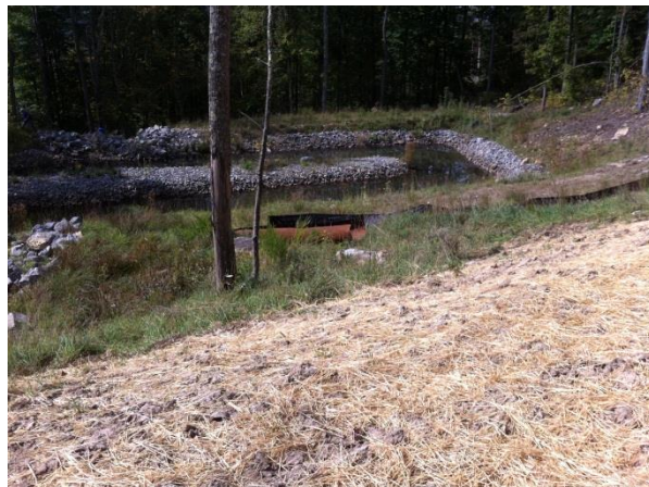
Figure 10: Inspection issues: note construction debris (such as discarded culverts) and remove it. Note any erosion of channels for AMD.
