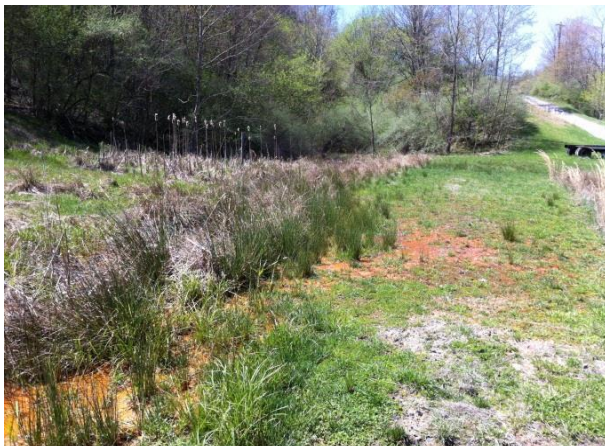
Figure 11: Inspection issues : channels may clog or back up, flooding adjacent ground. Drainpipes clog.
