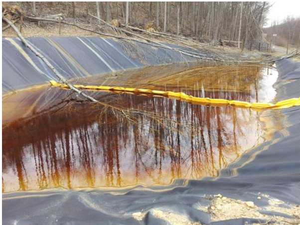
Figure 9: Inspection issues: note any logs that have fallen into any part of the project and clean them out. Note any evidence that water has flowed over an emergency spillway and maintain the project so that water flows through expected pipes and channels.
