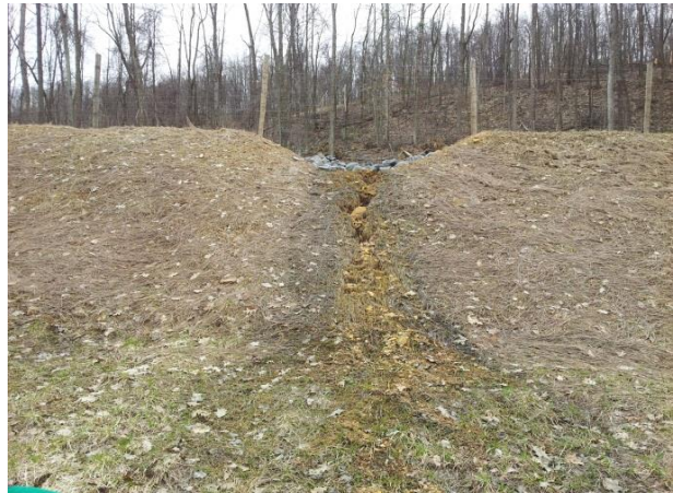
Figure 9: Inspection issues: note any logs that have fallen into any part of the project and clean them out. Note any evidence that water has flowed over an emergency spillway and maintain the project so that water flows through expected pipes and channels.
