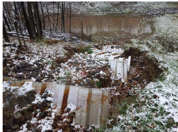
Figure 10: Inspection issues: note construction debris (such as discarded culverts) and remove it. Note any erosion of channels for AMD.
