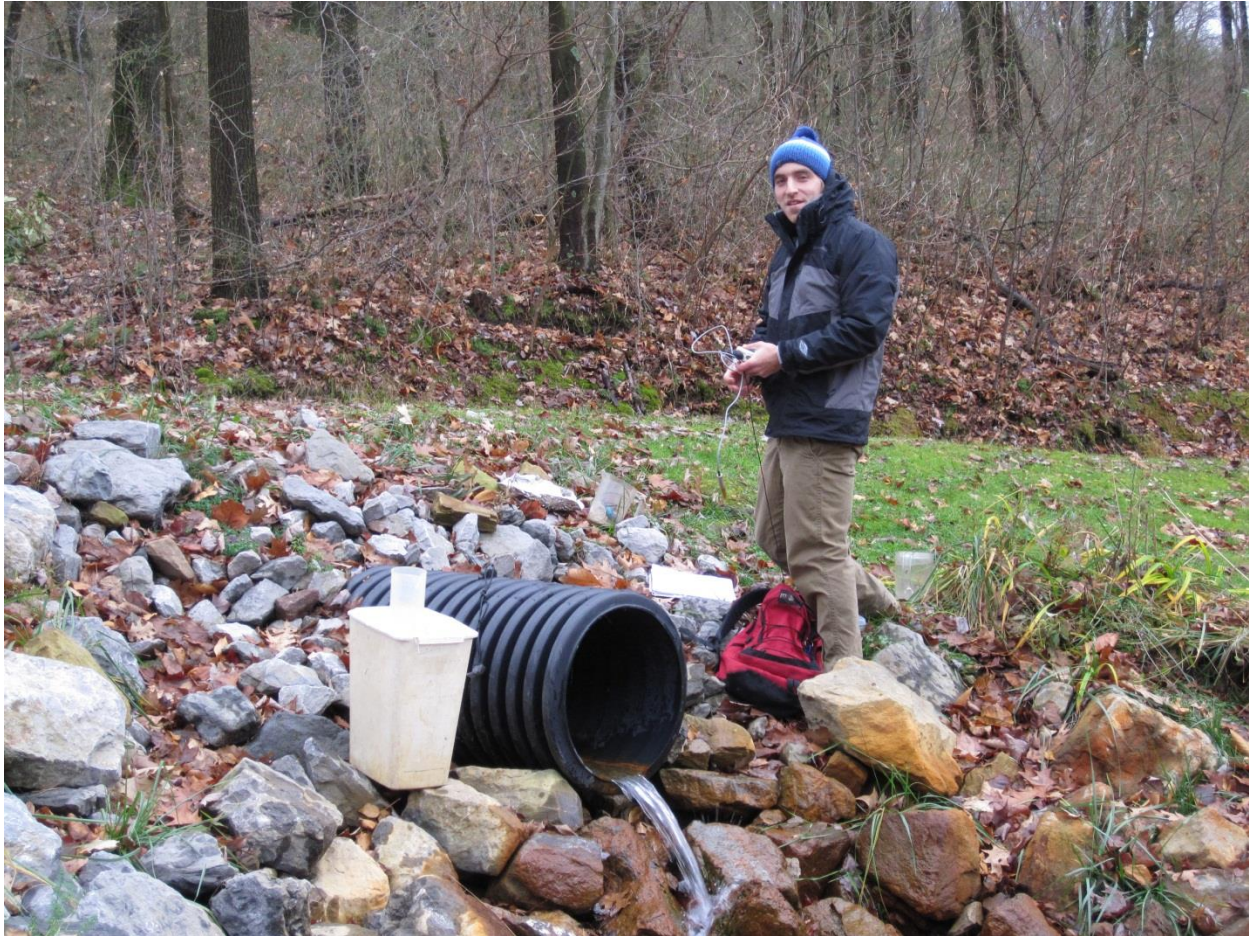
Picture 3: Brian Carlson monitors the discharge from a completed AMD remediation project. The drop beneath the culvert allows for measurement of flow with a bucket and stopwatch.
