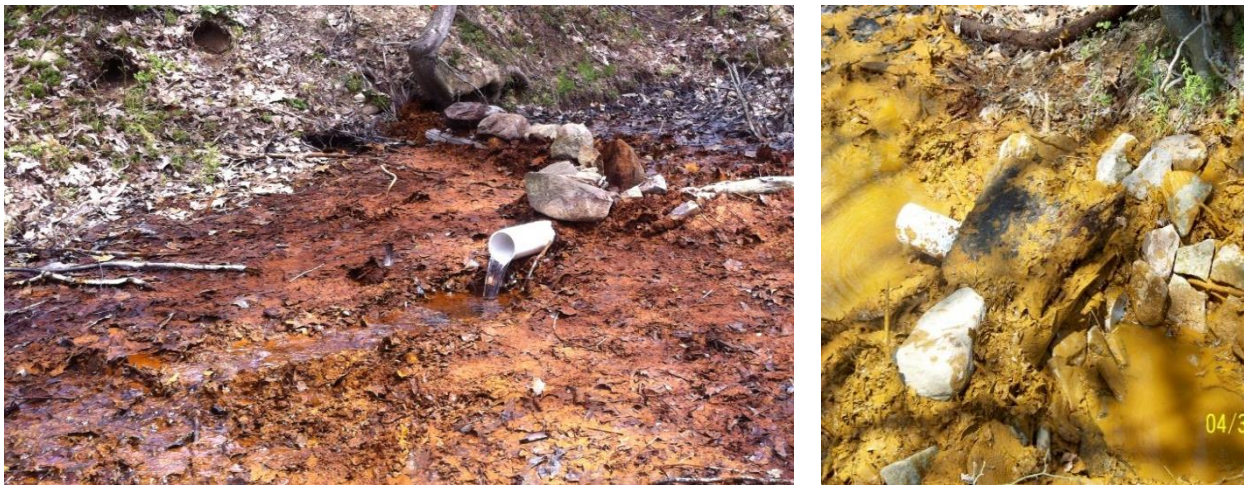
Figure 3: Left : Buckhannon River Watershed Association installed a flow pipe to measure flow at this seep; Right : soil and rocks are used to pool AMD so that it flows through the flow pipe
