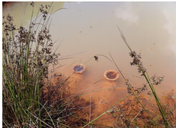
Figure 11: Inspection issues : channels may clog or back up, flooding adjacent ground. Drainpipes clog.
