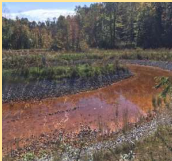
Low Flow Oxidation Limestone Channel
