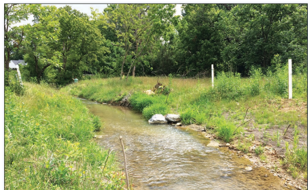
Figure 5. Lower portion of the restored reach.
