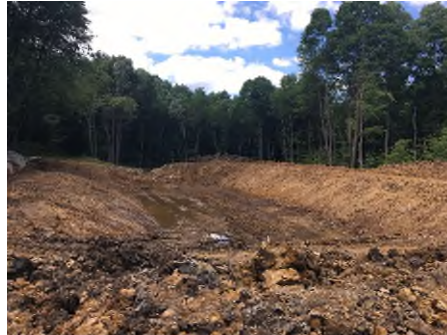
McElroy Seep - During Construction
