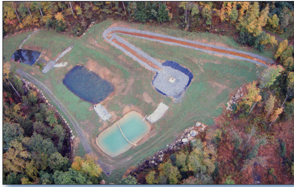
Figure 2. The North Fork Greens Run Railroad Refuse project passively treats AMD.
