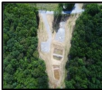
Auman Road: After
