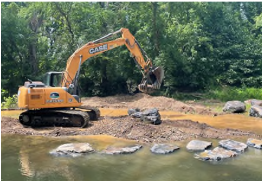
Boulder placement to enhance a stream in a watershed protection plan (WPP) priority basin.
