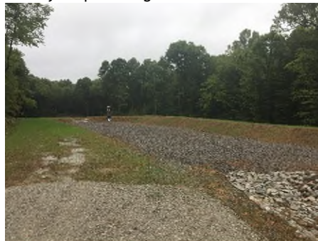
McElroy Seep - Post Construction
