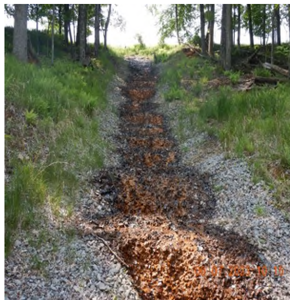
Figure 14. Photo of limestone terracing treating the Swamp Run 2 South seep.
