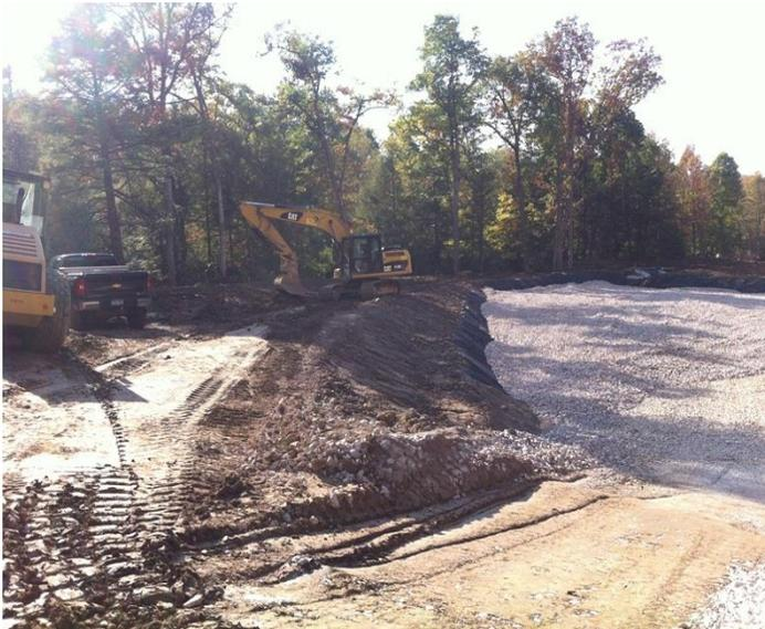
The photo shows a portion of the construction of a large leachbed in the lower section of the project.
