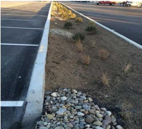
Water Quality Swale at the Foxcroft Mall in Martinsburg, WV
