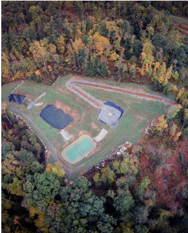
Aerial (drone) photo of Friends of the Cheat (FOC) North Fork Greens Run passive acid mine drainage treatment system.
