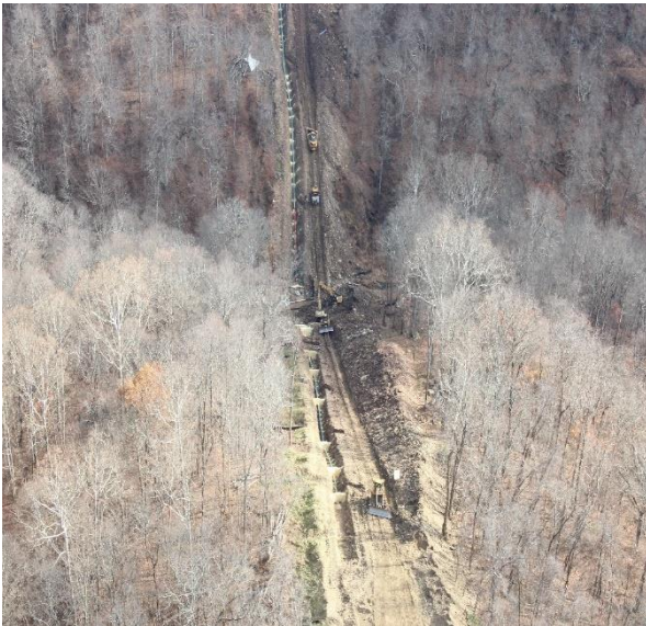
Picture 7 Oil and gas pipeline construction
