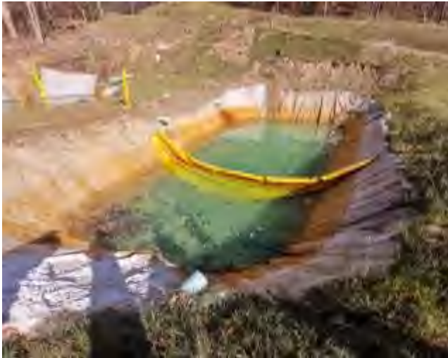
VH3 settling pond #2
