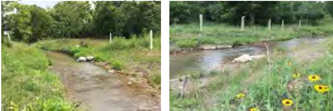
Stream restoration project site post-construction.
