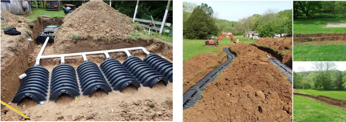
Figure 10. Septic work in the Browns Creek watershed.
