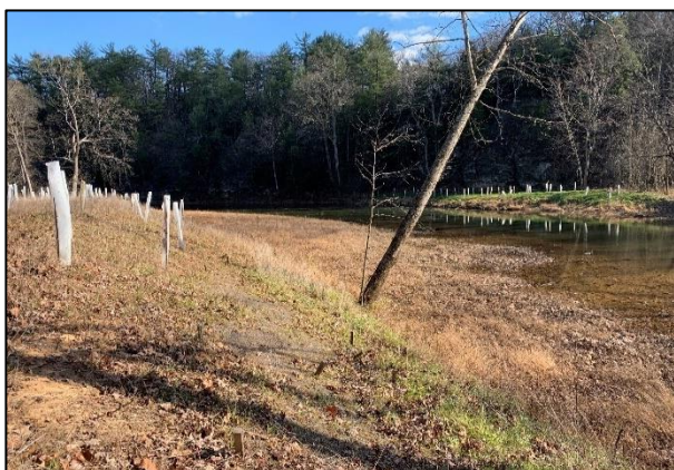
Back Creek stream restoration.
