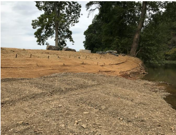
Regrading of bank on river left.
