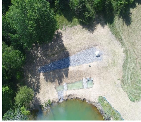
Beaver Creek at Auman Road Upper System Post Construction
