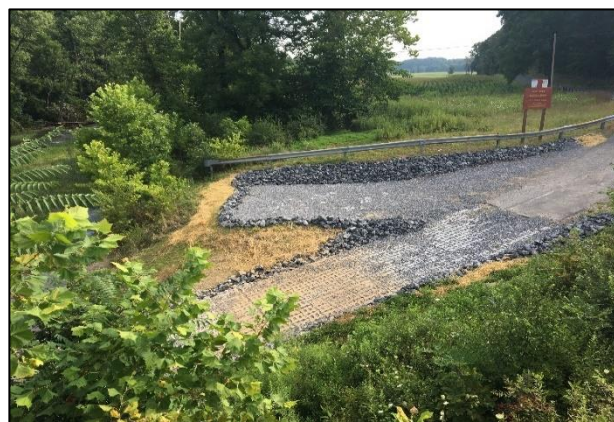
Porous paver installation at a public stream access on Back Creek.
