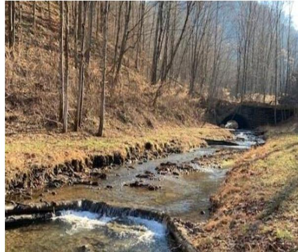
Stream structures being placed during the early phase of the Morris Creek restoration. Shortly after installation a heavy rain event occurred but the structures remained stable.
