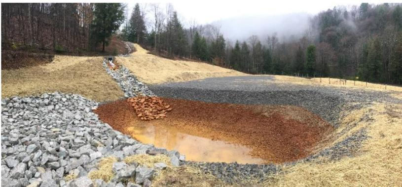
4,750 ton Auto Flushing Vertical Flow Pond filled with 90%+ CaCO<sub>3</sub> content limestone.
