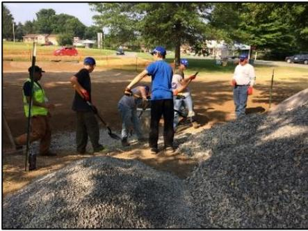
Another barren area along New River Drive in Beckley was contributing sediment to Little Whitestick Creek. This site was graded and revegetated in 2021. A rain garden was established to detain stormwater runoff from the front parking lots of the Raleigh County Convention Center. Some work was completed with assistance from a local boy scout troop. (Photos: 1-1A)
