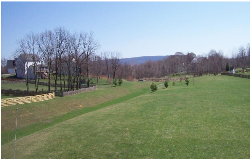
Figure 3. The drainage swale in Gap View Village, beginning in lower left of photo
