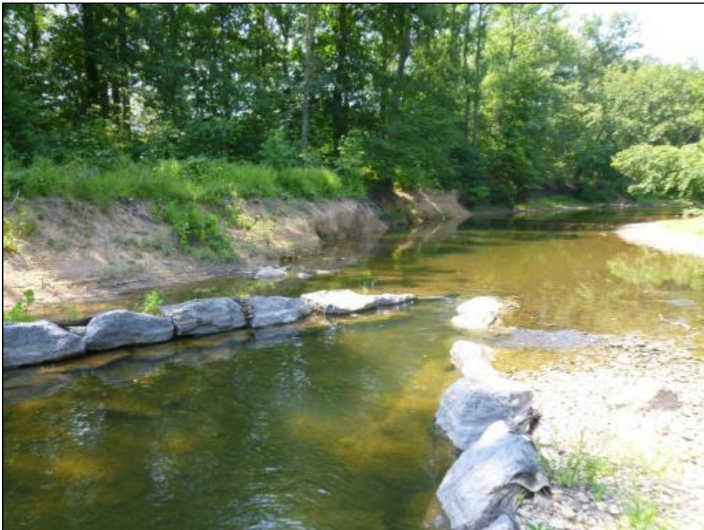
Photo 4. An existing in-stream rock structure (W-weir)
