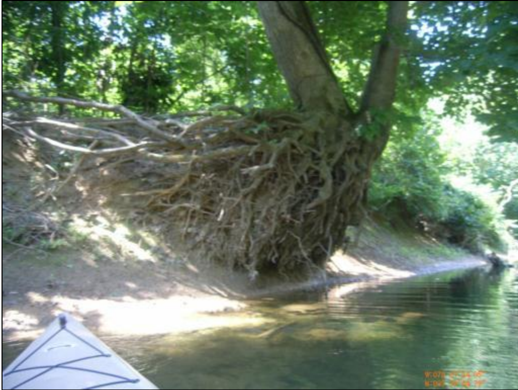
Photo 5. A highly eroded stream bank along Back Creek
