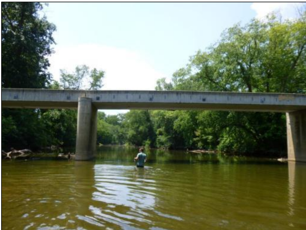
Photo 10. Example of a one lane bridge common in Back Creek.
