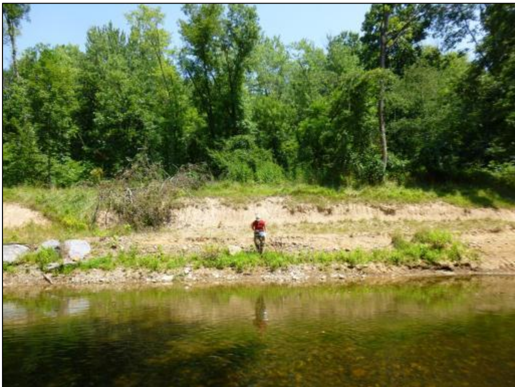
Photo 8. Terrace formation behind an existing NSD structure.
