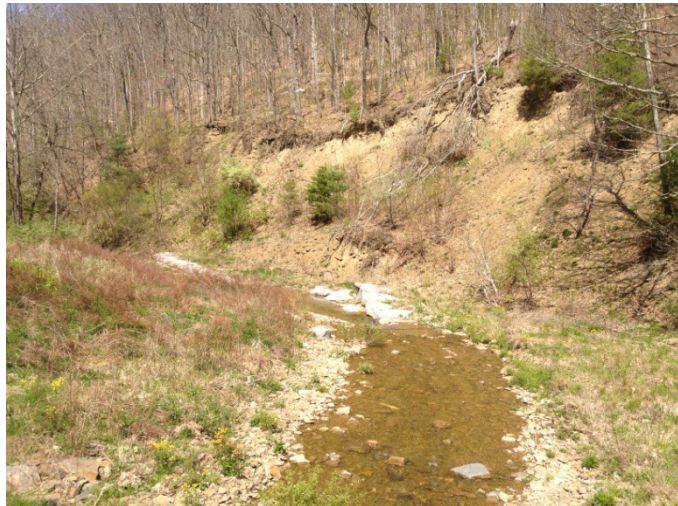
Figure 8: Knapp Creek: A cross vane redirects the current away from a vulnerable slip and creates a bench at the foot. Photo: Alvan Gale
