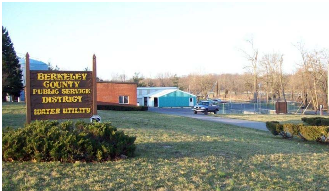
Figure 2. Berkeley County Public Service Water District's facility at LeFevre Spring, with a development construction project in the background.
