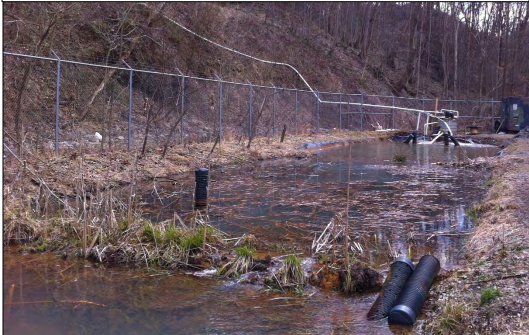
Figure 12 - Present state of Lower Mainstem treatment system; hillside seep has been rerouted to head of the treatment. It is piped through a hydro-generator and limestone diversion well before entering the system.
