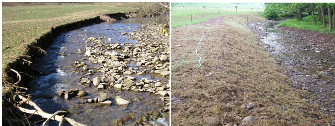
Figure 11: Kitchen Creek stabilization project, before and after
