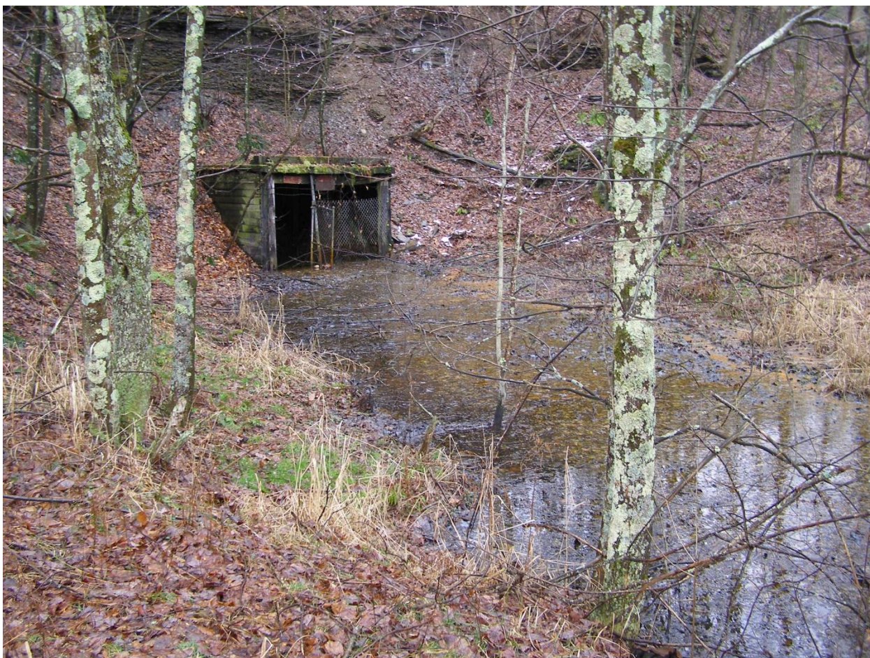
Figure 13. Portal 4 and its discharge.
