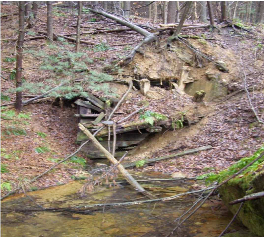
Figure 14. Portal 3 and its discharge.
