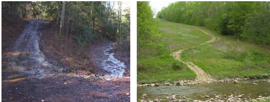
Figure 13. Reclamation of ATV impaired pipeline and abandoned gas well roads on the Left Fork of the Buckhannon.
