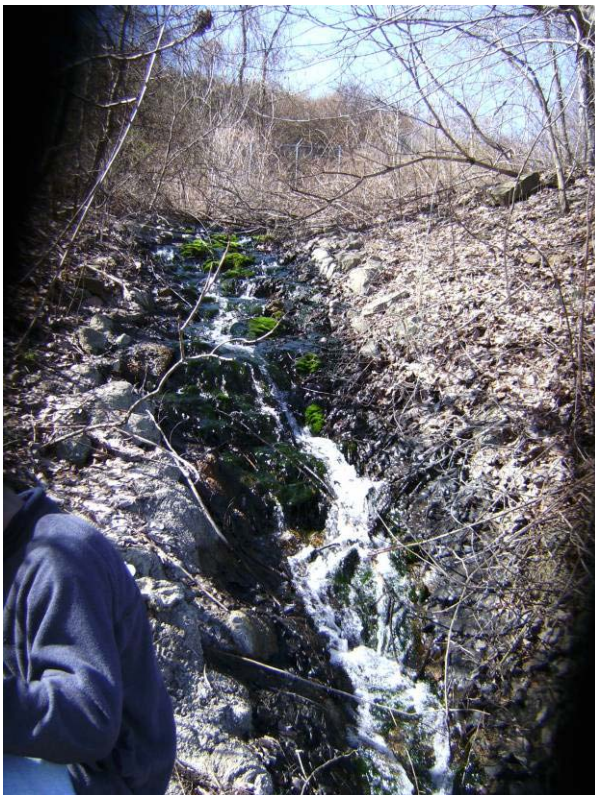
Figure 19: This photograph shows the Easton Left Portal discharge.
