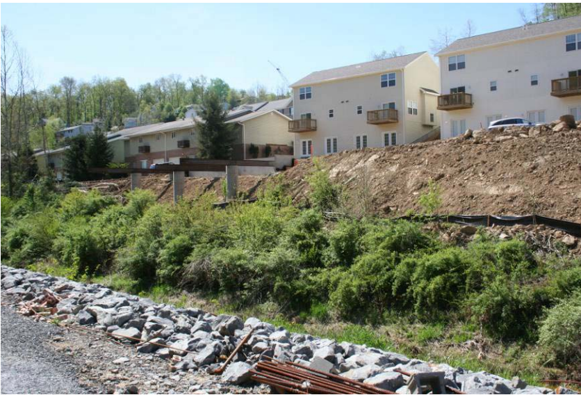
Figure 24: This photograph shows condominiums being built cantilevered over West Run.
