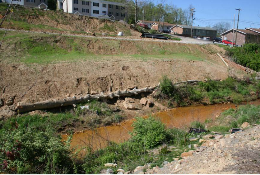
Figure 23: This photograph shows a tree being used as a silt fence.
