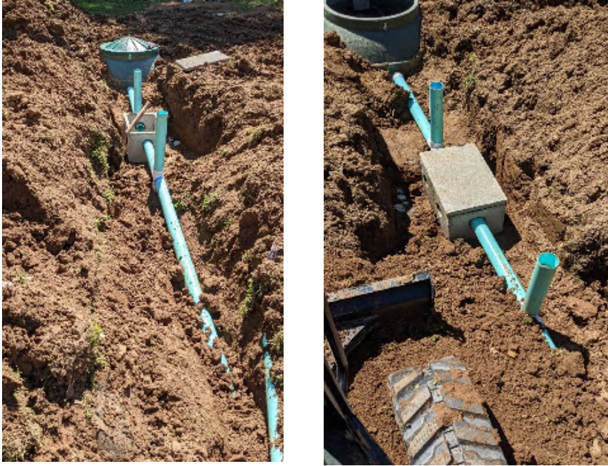
Figure 1. Examples of completed septic replacement.
