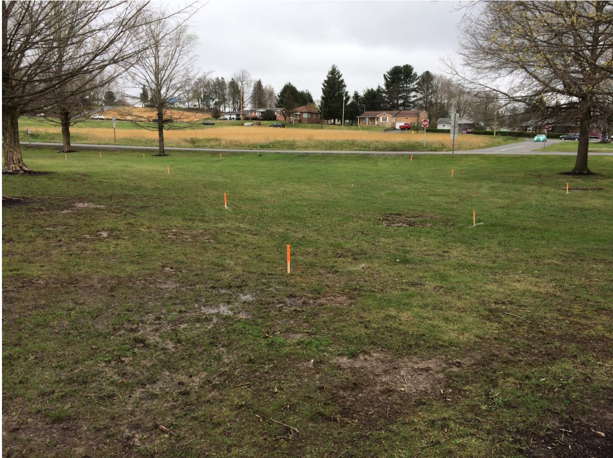
NPS 1586 pre-construction. Marking was done by the Executive Director and the Beckley Sanitary Board.
