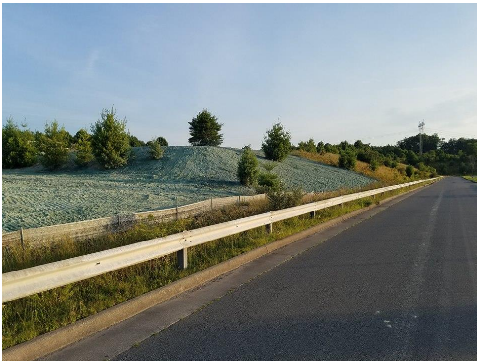
Project site on July 10, 2017 after hydro seeding.
