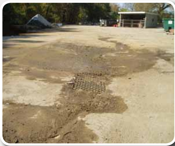
Public Works Yard
