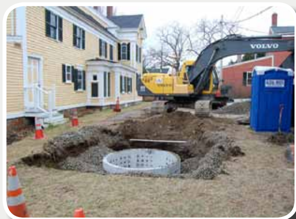
Disconnection with Compensatory Practice: Small-Scale Infiltration (Source : http://www.brickstoremuseum.org/campaign_timeline.shtml )
