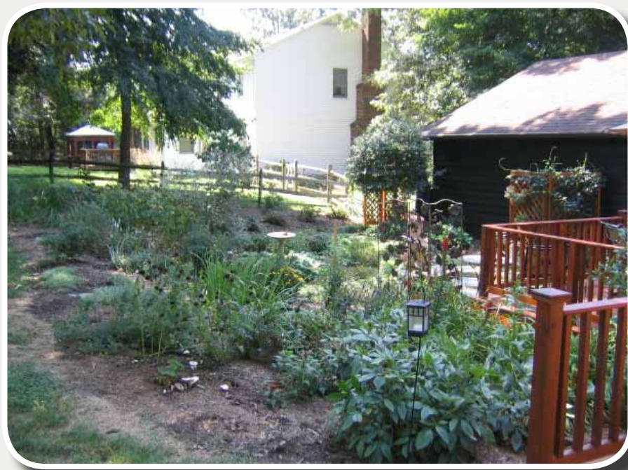
Figure ID-7.A backyard rain garden that treats rooftop runoff
