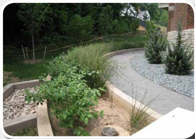
Adjacent to building to catch roof runoff
