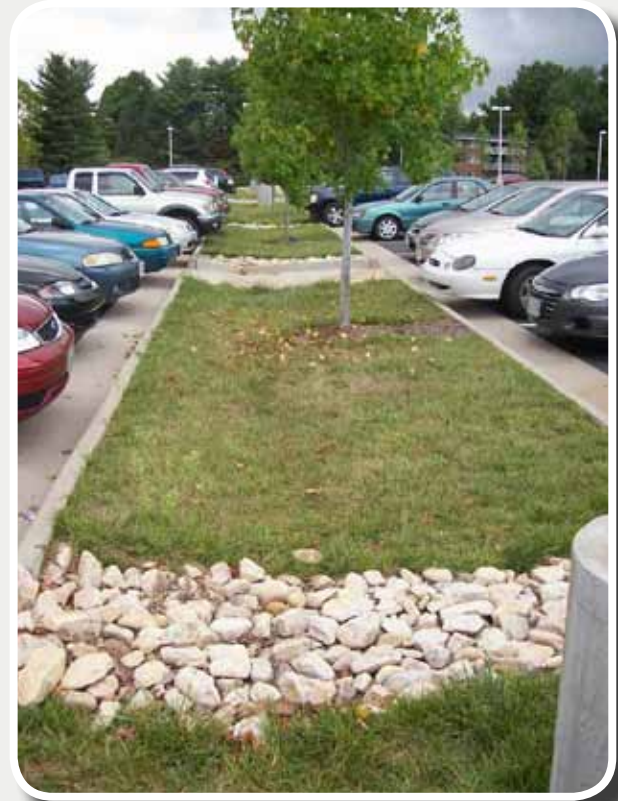
Turf-covered Water Quality Swale with curb cuts and stone pre-treatment
