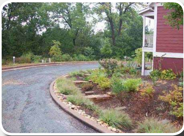
Water Quality Swale with check dams along roadway
