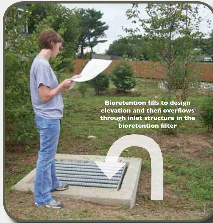
Figure BR-12. Top: Example of an off-line design where only the design volume goes to the Bioretention cell. This can also be accomplished with diversions or flow splitters upgradient from the cell. Bottom: Example of an “on-line” design where all the flow enters the Bioretention, and flows that exceed the design elevation overflow into a structure within the practice.
