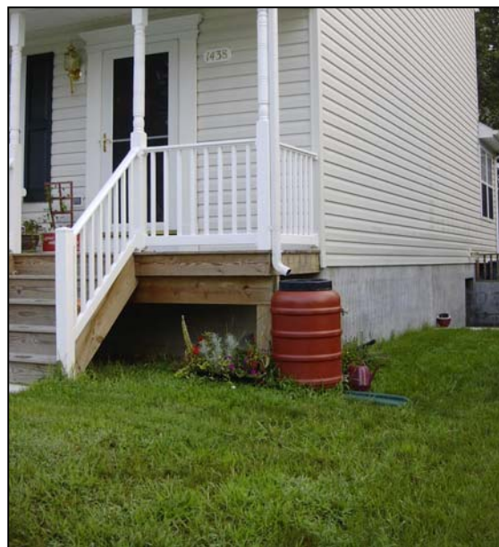
Figure 1: Installed Rain Barrel
