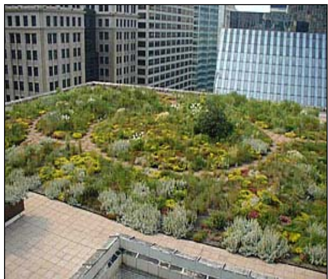
Figure 1: Green Rooftop on Chicago’s City Hall Source: Roofscapes Inc. www.roofmeadow.com
