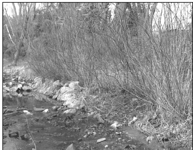
Figure 1: Fascines installed behind a boulder revetment
