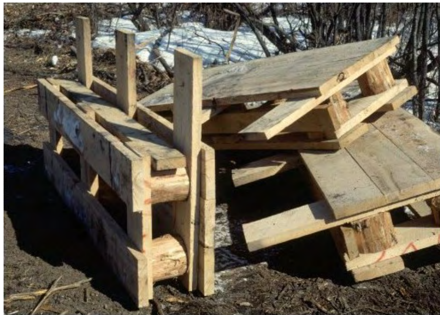
Figure 1: Assembled lunkers prior to installation Source: Minnesota DOT
