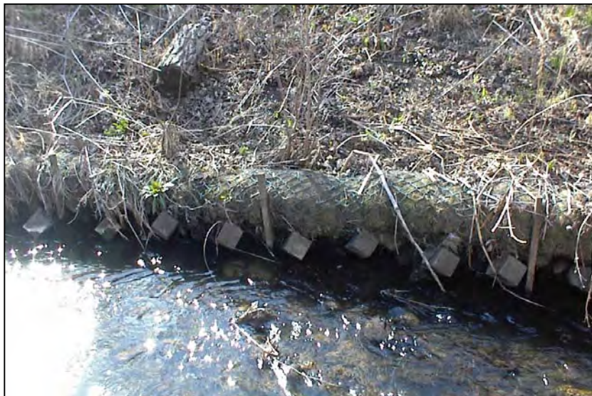
Figure 1: A-jacks installed beneath coir fiber logs
