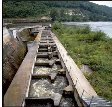
Figure 1: Vertical slot fishway
