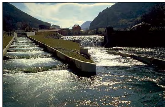
Figure 3: Pool and weir system on the Dordogne River (France)
