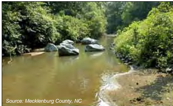
Figure 1: Boulder cluster installed in a stream
