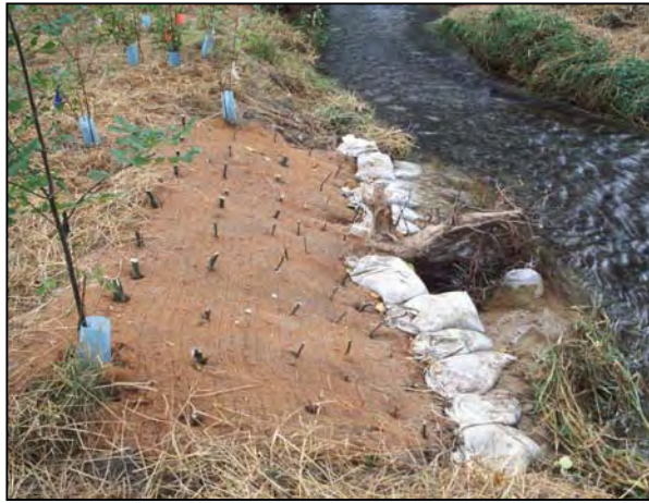
Figure 2: Biodegradable coir fabric with live stakes
