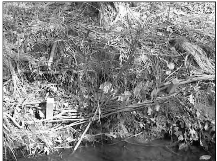
Figure 2: Fascines installed along a streambank
