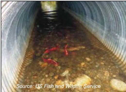
Figure 2: Channel simulation – embedded culvert Orchid Lake, Alaska
