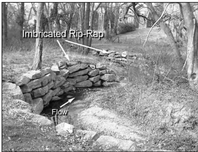
Figure 1: Imbricated rip-rap revetment protecting utility infrastructure
