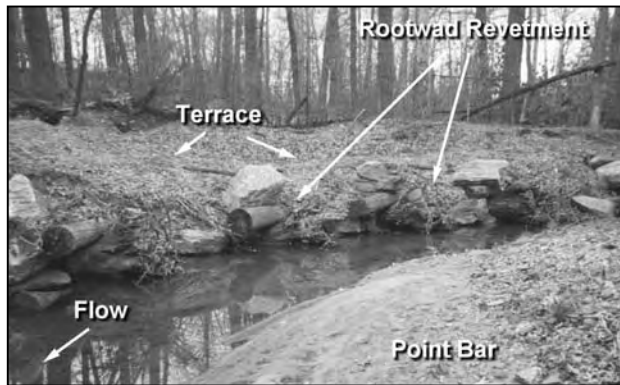
Figure 3: Stable rootwad revetment along an urban stream
