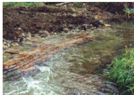
Figure 3: Newly installed lunkers Source: Vernon County, MI LWCD
