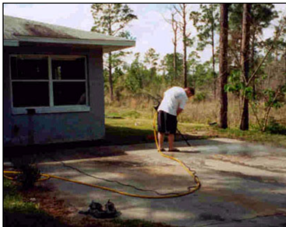
Figure 1: Power Washing of a Driveway
