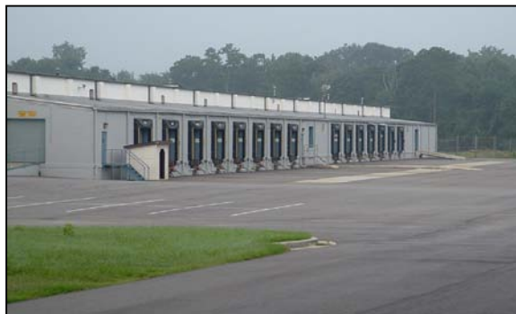
Figure 1: Loading/Unloading Area of Warehouse
