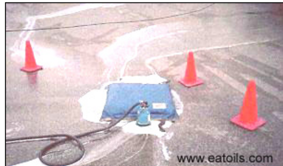
Figure 2: Storm Drain Cover Used when Washing with Soaps
