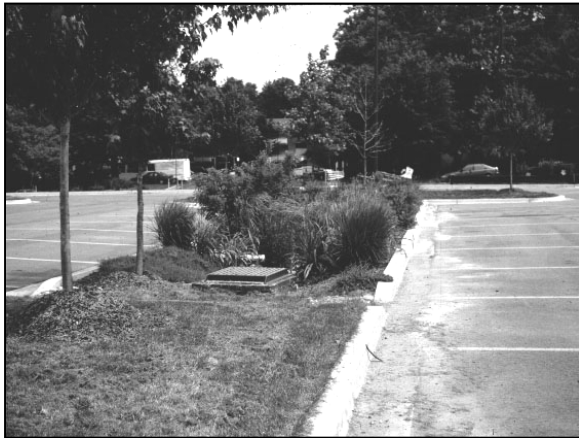
Figure 2: Parking Lot Island Turned Bioretention Area
