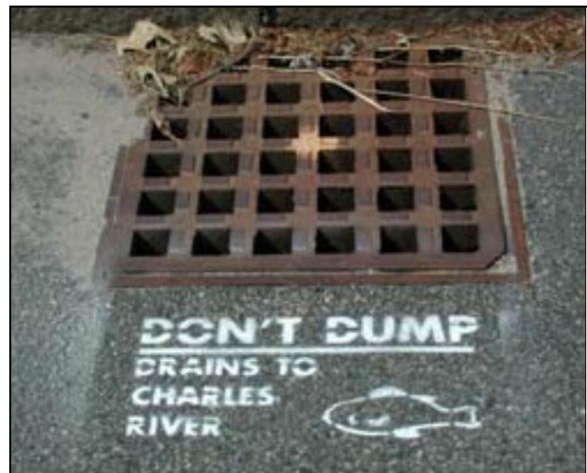
Figure 1: Storm Drain Marking
