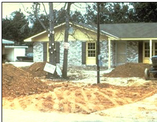
Figure 1: Soil Compaction During Remodeling
