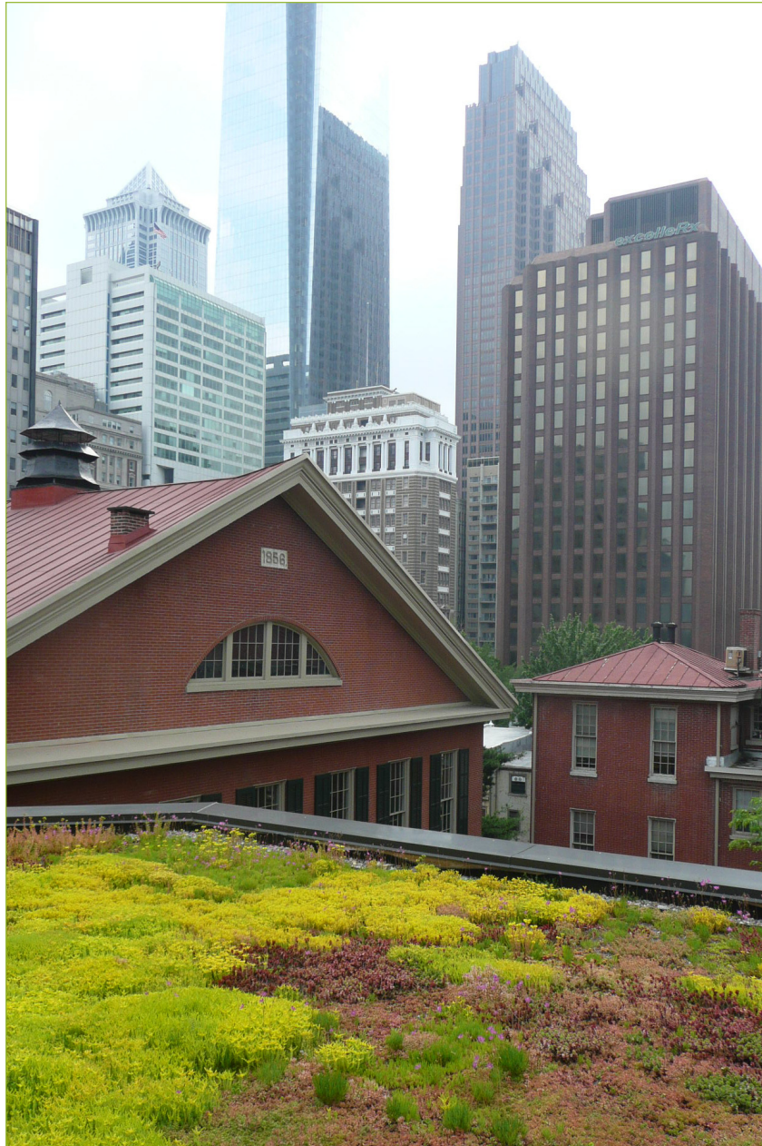
A green roof located on the Friends Center in downtown Philadelphia, Pennsylvania provides stormwater management capacity and adds aesthetic value to this dense urban environment.
