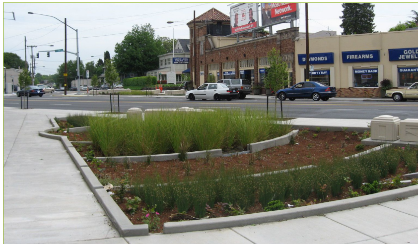
Street retrofits can integrate green infrastructure, like this bioswale along Sandy Boulevard in Portland, Oregon, into standard roadway maintenance and upgrades.
