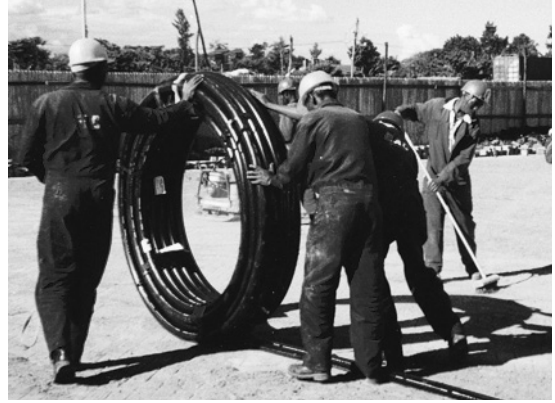
Figure 4: Uncoiling Pipe
