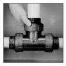
NOTE: Tighten by hand only until coupling bottoms out into fitting. Do not continue to tighten the nut once the coupling has stopped.
