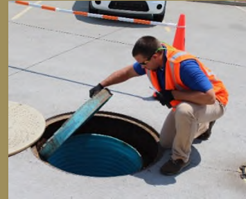
Inspecting a containment sump
