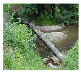
portion of the pipe and its diameter. The same applies to any pipes running parallel to the stream channel along the stream bank. Look closely to see if a given pipe shows any signs of fracture, or has any apparent discharge leaking from a fracture or natural joint.
