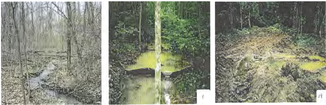
The 1 st photo is Harper Run above the track; the second photo, silt fences placed directly into the stream creating a sediment dam; in the 3 rd photo it is difficult to distinguish between land and water, in this case dirt was piled into the stream during trail construction.
