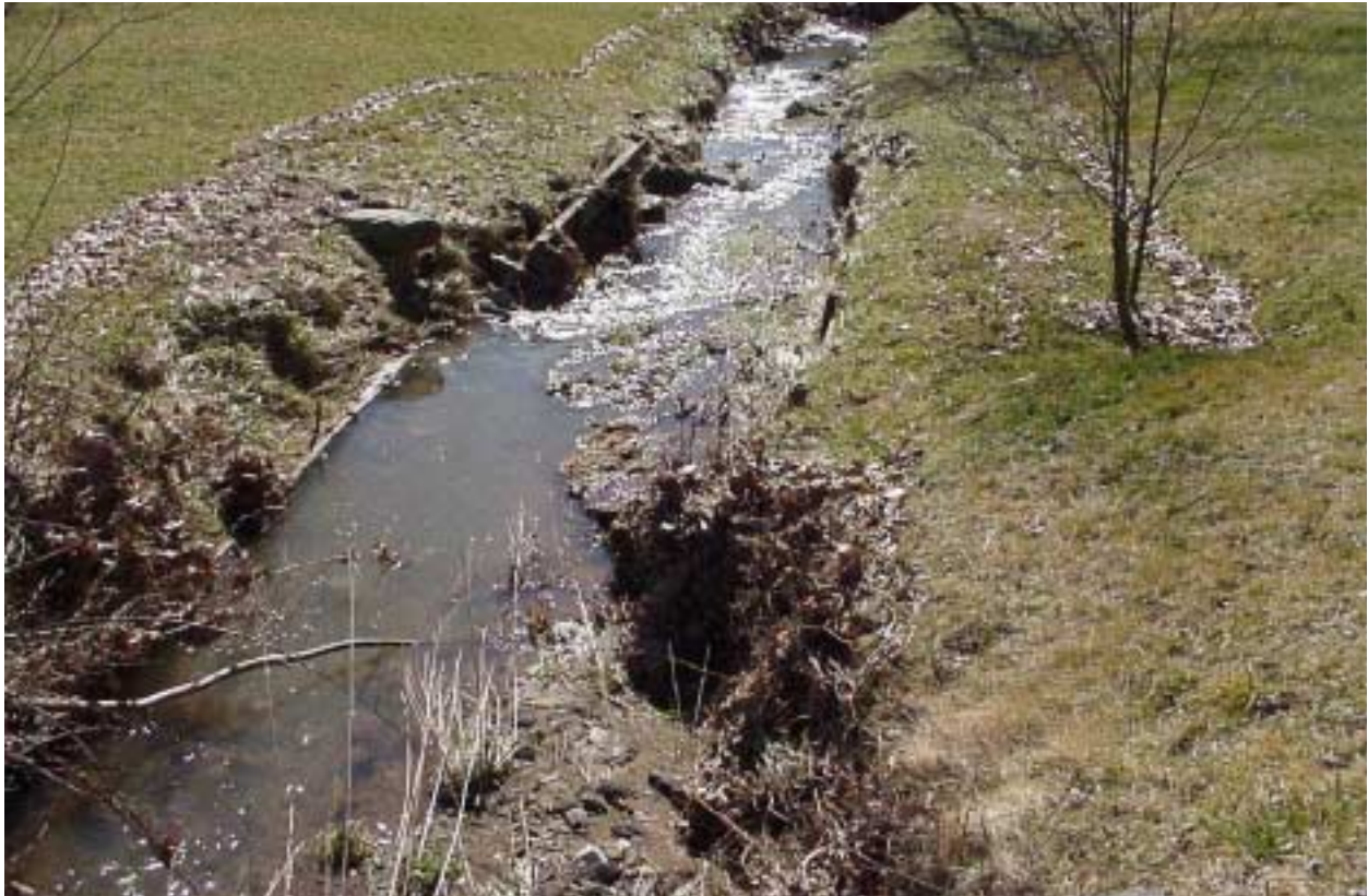
HIGH WATER MARK LEFT IN YARD ON TRIBUTARY OF KANAWHA TWO MILE
