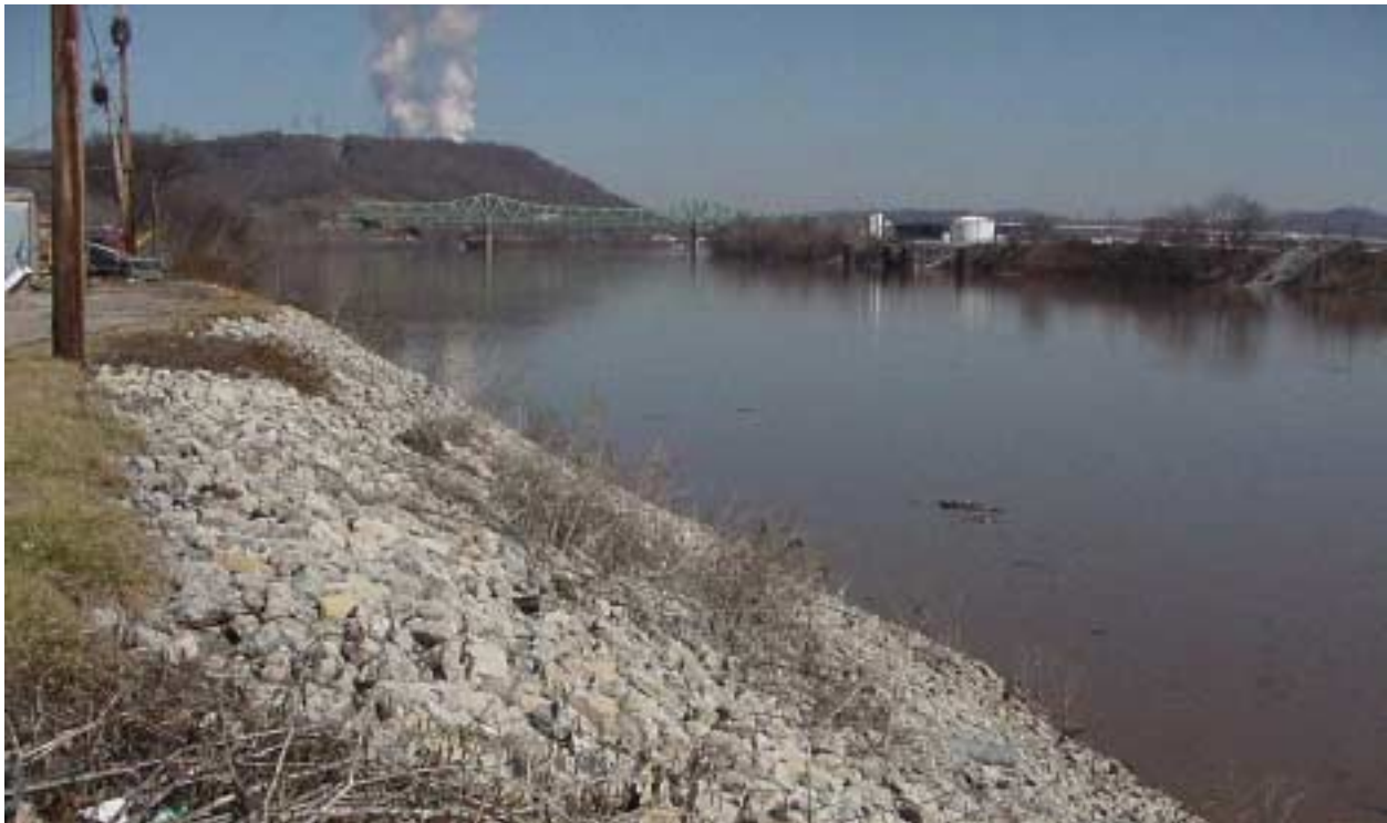
BANK STABILIZATION ALONG KANAWHA RIVER NEAR ST. ALBANS
