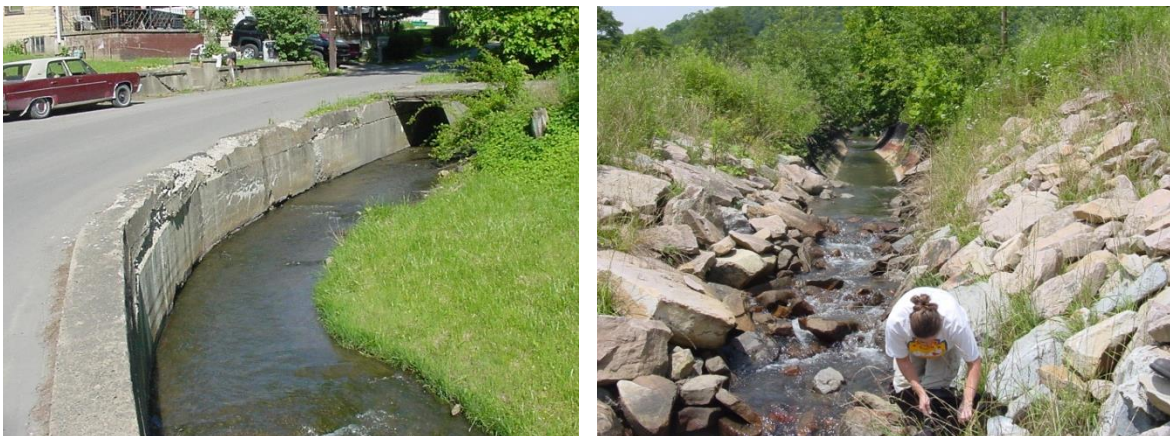
Figure 2-32. Examples of varying degrees of Channel Alteration (concrete channel on left and rip/rap channel on right).
