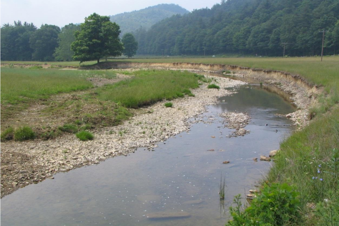
Figure 2-39. Example of an unstable bank. Note the lack of trees (and roots) to provide soil stabilization.
