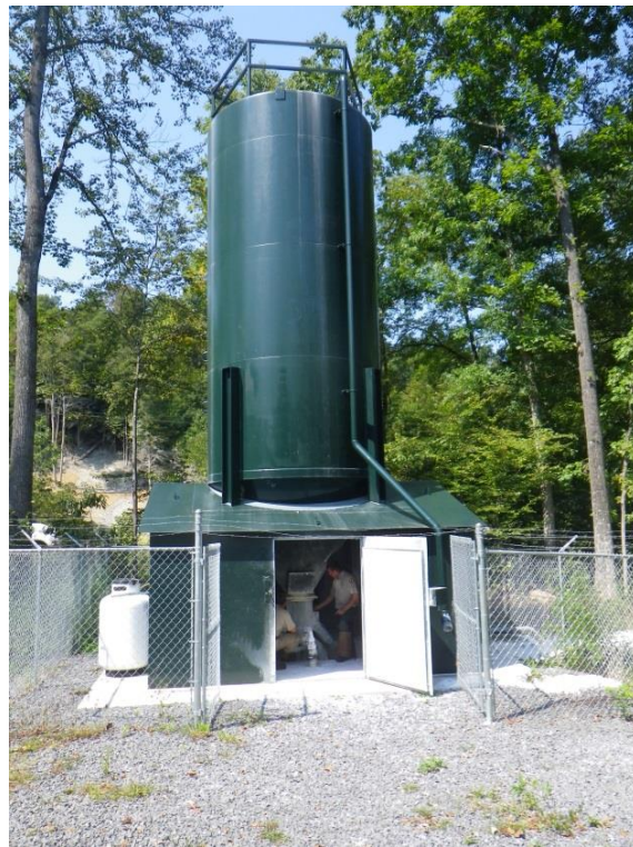
Figure 19-Typical design of an AMD treatment station.
