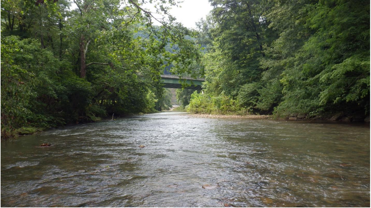
Figure 16-Looking downstream at mile 5.7.
