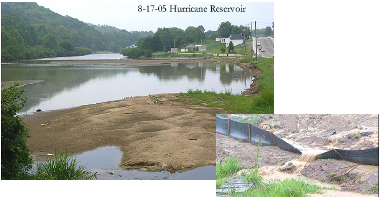
Figure 5.3 Sedimentation of the Hurricane Reservoir - A Factor that Exacerbates Low Flows and Flood
