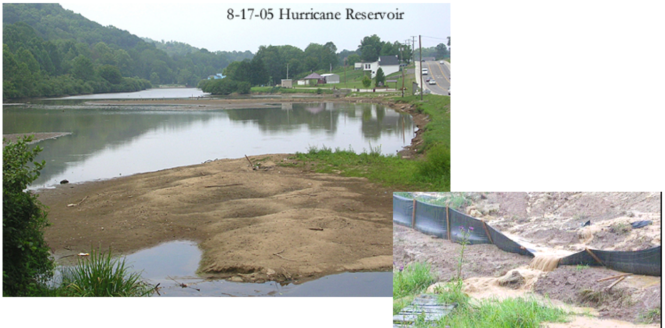
Figure 20. Sedimentation of the Hurricane Reservoir - A Factor that Exacerbates Low Flows and Flood
