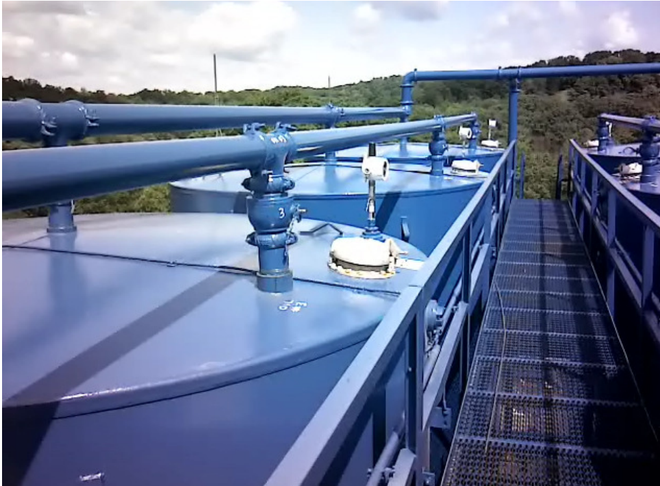
Condensate Tank Thief Hatch Vapor Leaks
