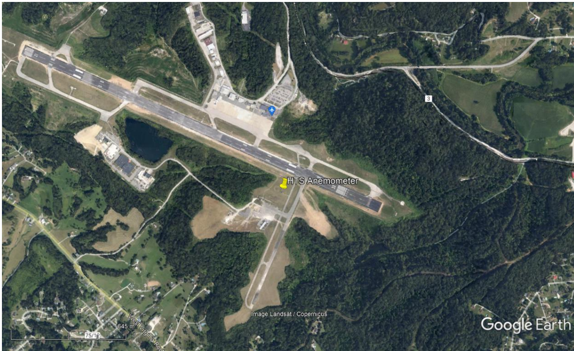
Figure 4-1. Aerial Image of Huntington Airport
