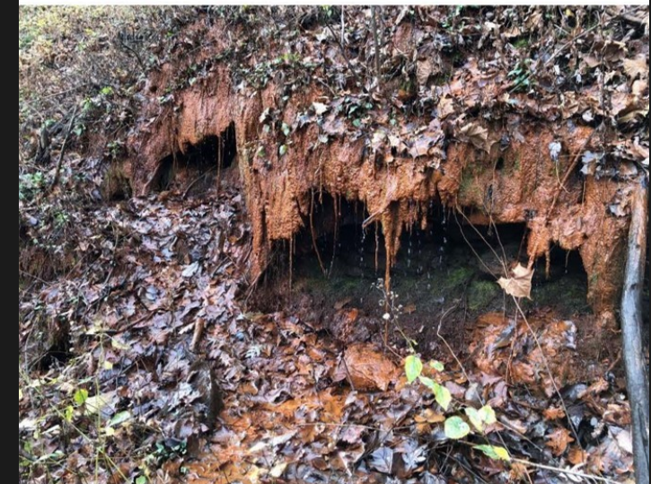
Collapsed and Draining Entry-Top of Main Slide
