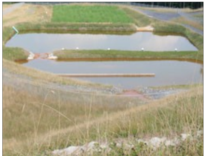
Passive system is successfully treating mine drainage
