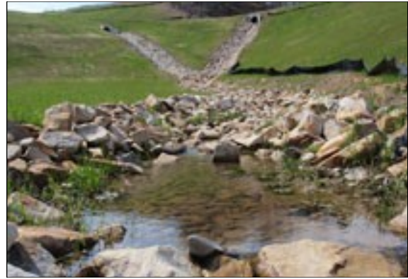
Stream channel design reduced acidities by one-third
