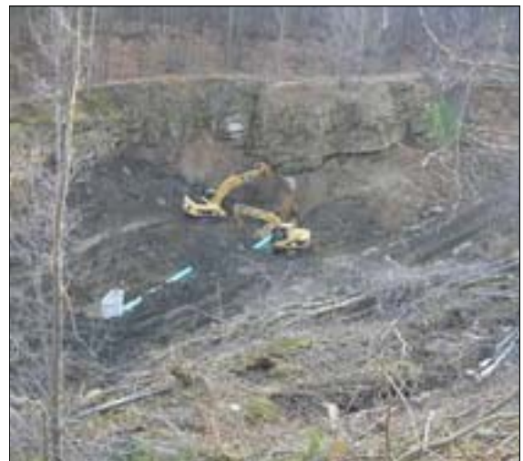
Exposed high wall
