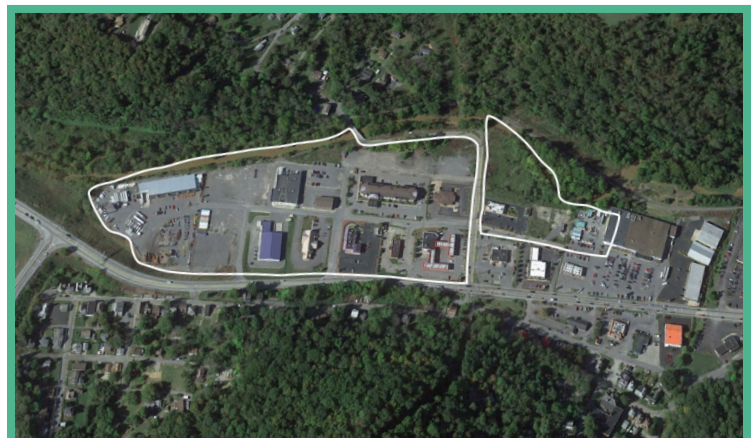
A cap (clean soil and asphalt pavement) was placed in certain areas, and a land use covenant was recorded with the property deed to prohibit residential use of the property. Today, the site is populated with several commercial businesses, including banks, restaurants, retail stores, and a hotel.
