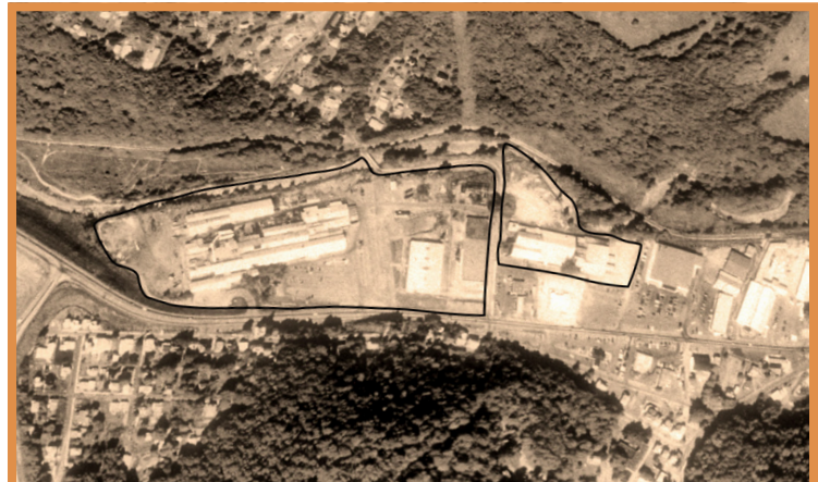
This 30-acre site was previously home to a tin plating mill, plate glass manufacturer, and metal and plumbing parts manufacturer, until all operations ceased and the site was abandoned in 1995. The property participated in the WV Voluntary Remediation Program to determine environmental impacts from previous site uses and restore the property for redevelopment.
