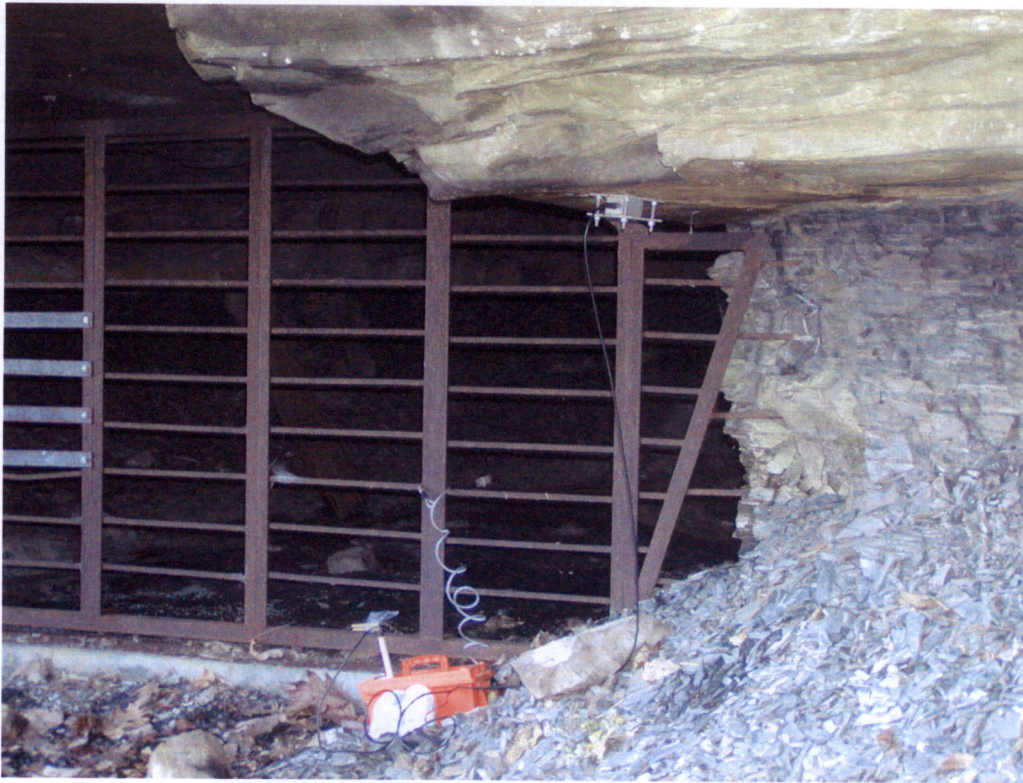
Figure 4 – Geophone Bolted to Roof of Portal 2A
