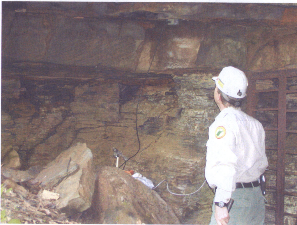
Figure 5 – Geophone Bolted to Roof of Portal 2D
