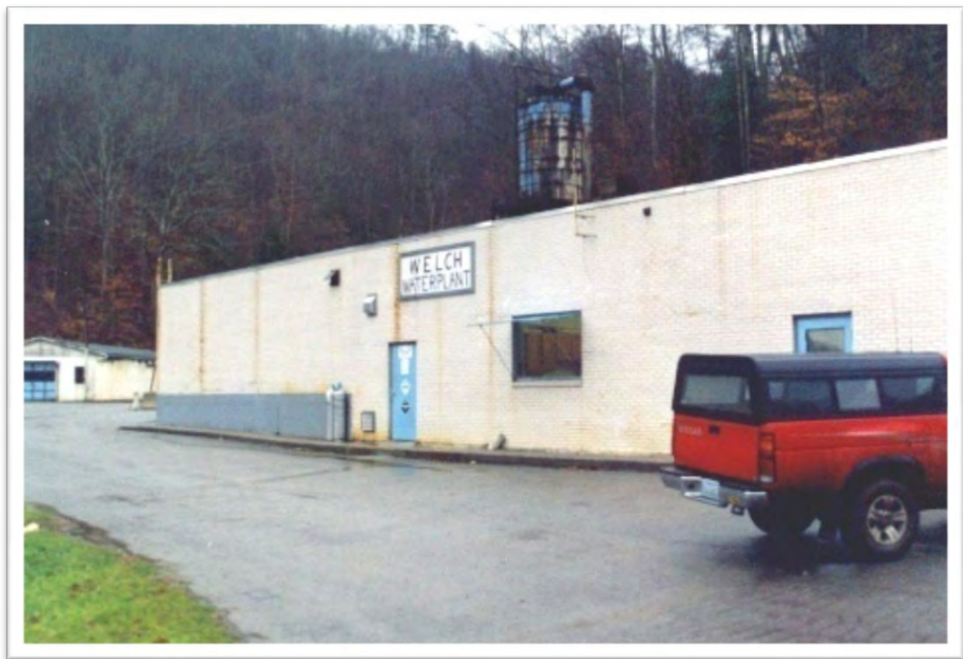
Figure 37 Welch Water System (Photo from DHHR files).
