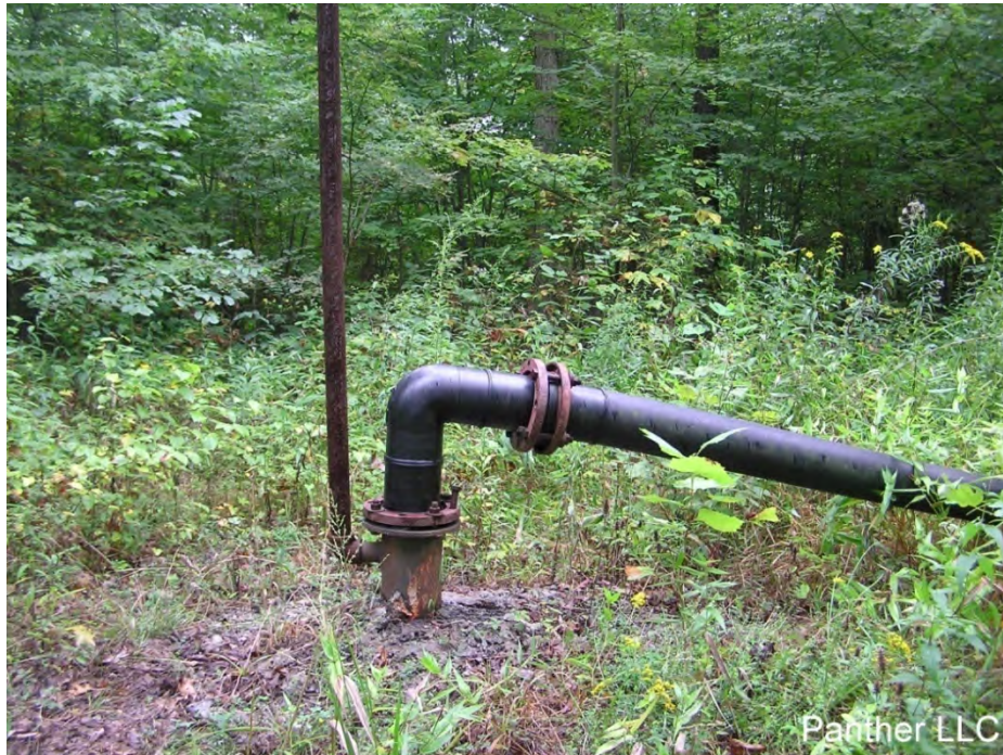
Figure 8- Inactive Panther slurry pipeline into injection hole
