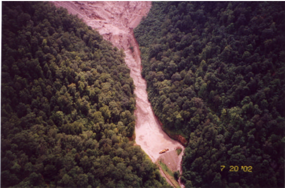
Picture 15 – Face erosion that flowed through the sediment pond and down Lyburn Hollow.
