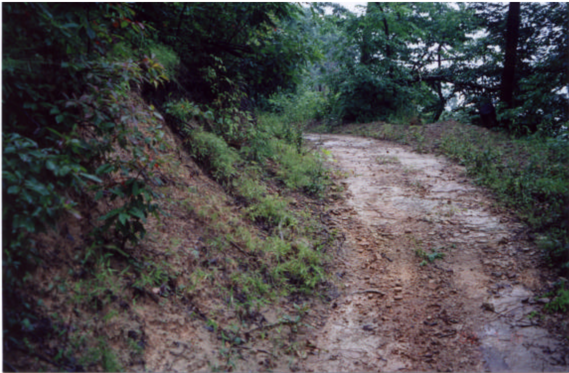
Picture 5 – Abandoned skid road with outer berm in place showing erosion to bedrock.
