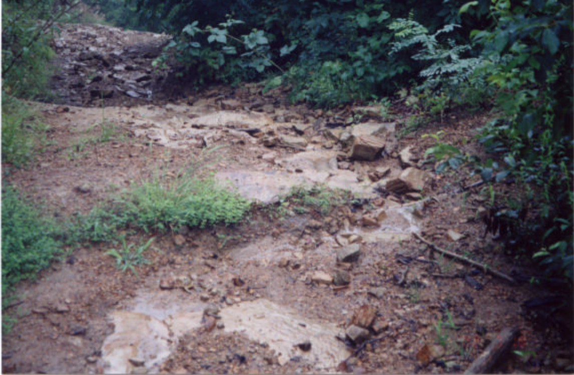
Picture 4 – Flow channelization and erosion through a waterbar on a skid road.
