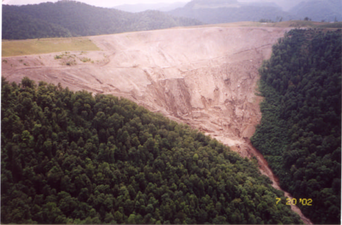
Picture 13 – Lyburn durable rock fill showing face erosion.
