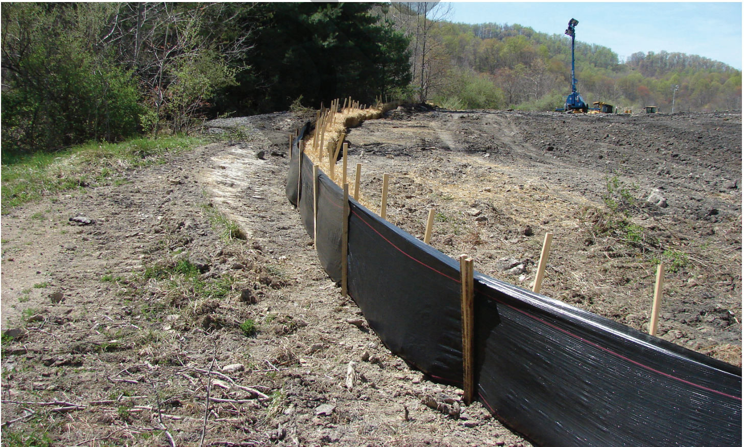
Figures II-7 Sediment Barrier Examples
