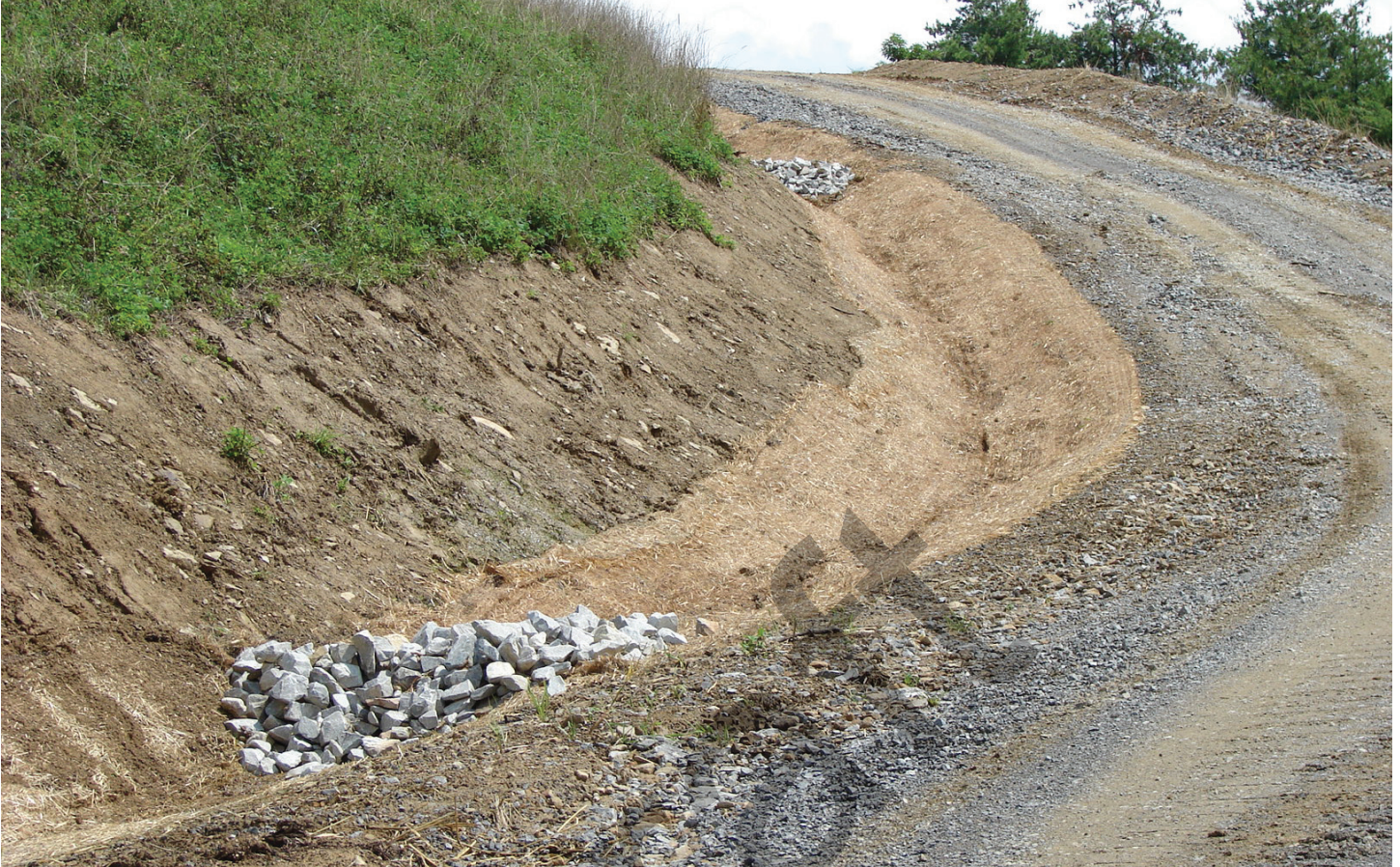
Figure II-5 Rock Ditch Check Dams Example
